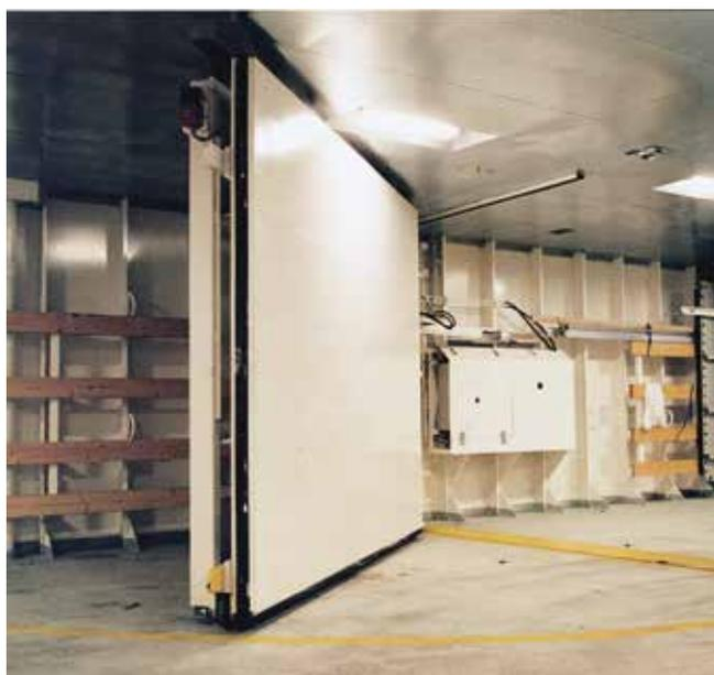
A number of solutions for flood prevention are available including the side-hinged and sliding door, which is fitted with a sliding end section. With this solution, the door is stowed at the side of the opening and can swing through either 90 or 180 degrees depending on ship design and operator needs.
